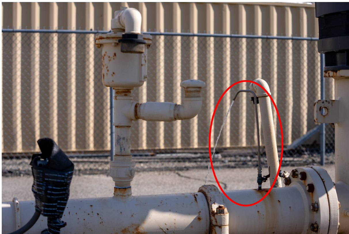
Example of a sample port location close to a well head, circled.
